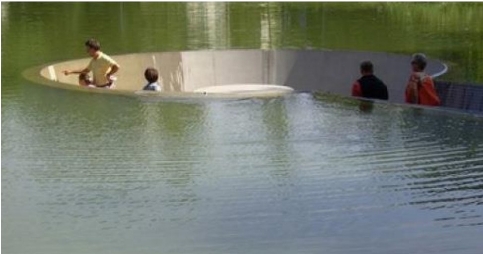
OBSERVATION DECK. VOCKLABRUCK, AUSTRIA. WESTPOL
