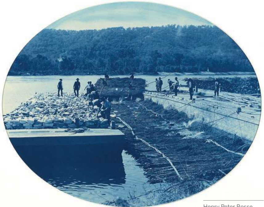
Henry Peter Bosse, Construction of Rock and Brush Dam, L.W. , 1891, cyanotype, 10 7/16 x 13 1/8, National Gallery of Art, Washington, Gift of Mary and Dan Solomon
