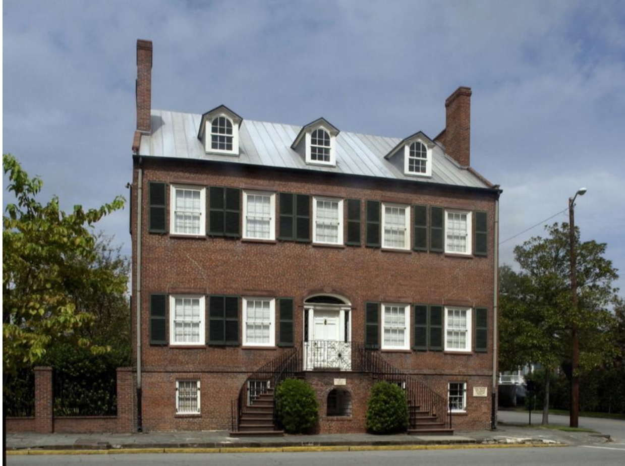
Davenport House (Savannah, Georgia), 1820
